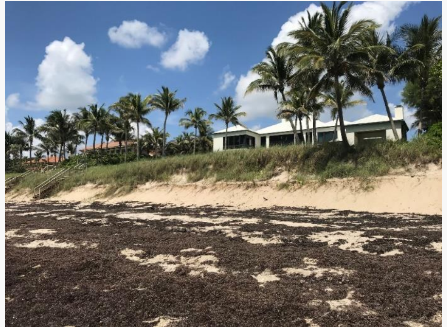
Areas of Active Erosion
