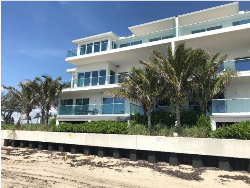
Areas with Poor Engineering
